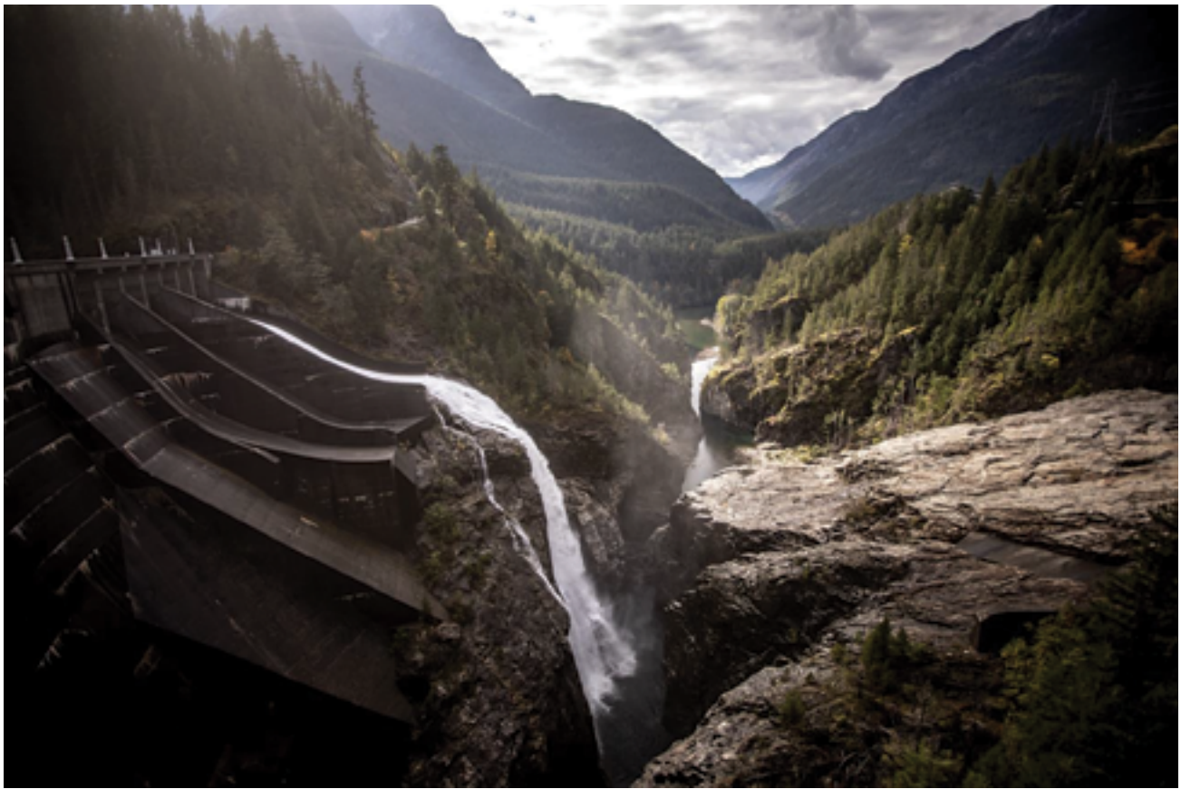
Aerial view of the Diablo Dam. Image courtesy of HDR.
