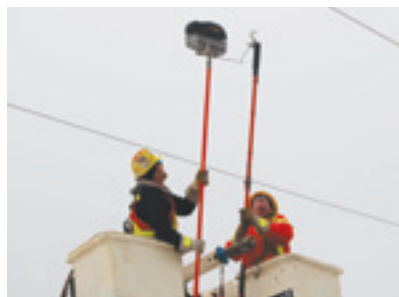
Live line installation of DLR conductor monitor in Cold Lake, Alberta, Canada
