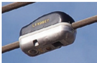
Next generation DLR conductor monitor
