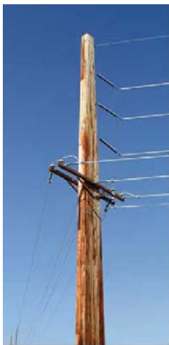
Unguyed full-tension dead-end laminated pole.
