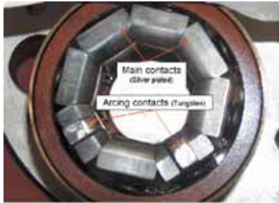
Fig 7 Tulip contact in oil circuit breaker
