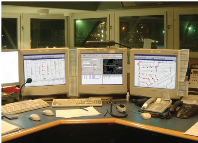
Figure 2 – Consolidating disparate data from multiple applications into one common operating picture is key to managing the deluge of data from smart grid technology. This centralized command-and-control center allows one operator to manage grid operations through a single application on just a few screens. When not consolidated, a utility may be using 7-10 monitors in separate locations with multiple applications.
