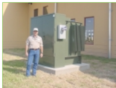
Figure 4: MeterSmart Technician Billy Echols prepares to download 30 days of interval data from the mass storage meter mounted on the side of the padmount transformer outside a Sharyland commercial facility. The data will be e-mailed in HHF format to UDRI/MeterSmart for input into the data processing software system.
