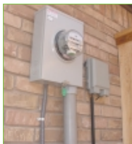
Figure 3: Common utility trenching simplifies installation of phone-based AMR solutions. The AMR module is installed under the meter glass and connected to the phone line at this Sharyland residence.
