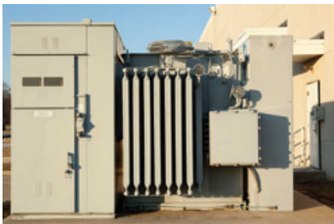
Figure 2. Most electrical switchgear is designed for operation in relatively benign outdoor environments. Classic failure points include bolts, door gaskets and other areas where liquid or particulate ingress can destroy the switch or breaker circuitry.
