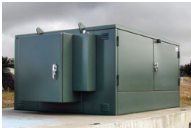
Figure 3. Trayer 3805 series medium-voltage electrical switchgear installed by Central Lincoln PUD at the NOAA Pacific Fleet Headquarters provides high-speed automatic transfer and double-sided access. The unit's corrosion-resistant 304 stainless steel enclosure requires no maintenance and prevents rusting in harsh marine and inland storm environments. Note placement of boulders as a landscape barrier to protect the pad from vehicular traffic.
