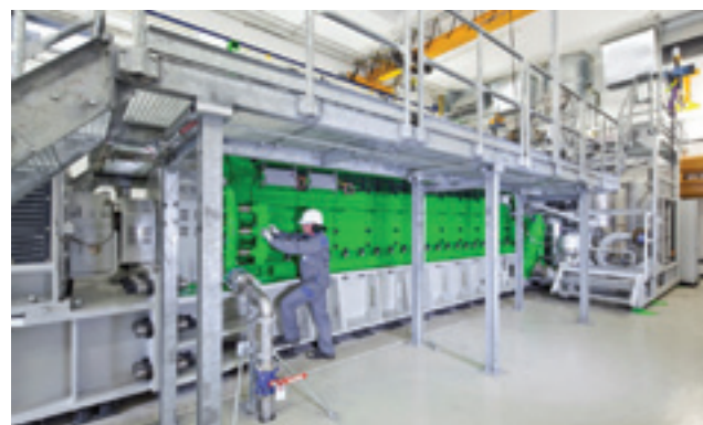
GE's 10 MW class J920 FleXtra engine is part of the Stadtwerke Rosenheim municipal cogeneration plant in Germany
