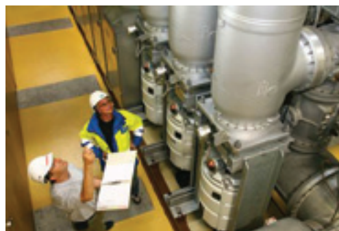
Fig 1: La Foretaille GIS substation in Switzerland. The older-generation circuit breaker type SN was replaced by an ELK SP2-1 with AHMA drive.
