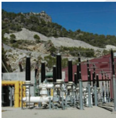
Fig 3: La Muela GIS substation, Spain. The HKA8 drive was replaced with the HMB8 on SL3-2 circuit breaker.
