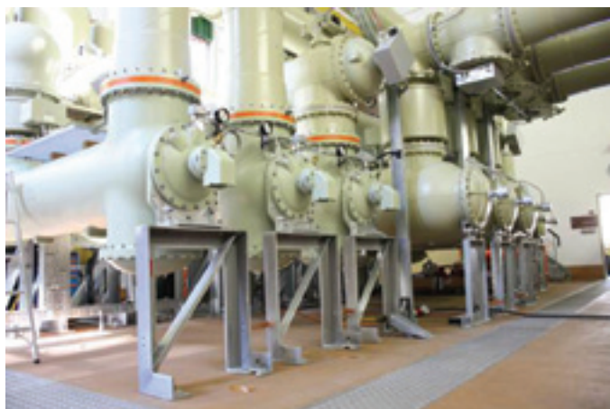
Fig 2: Filisur GIS substation, Switzerland. The SL3-2 circuit breaker and HKA8 drive were replaced by a single chamber SP3-1 circuit breaker with HMB4 drive.
