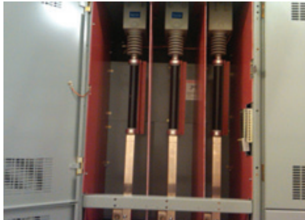
Figure 2 – R-C Snubber Installed at Customer Facility
