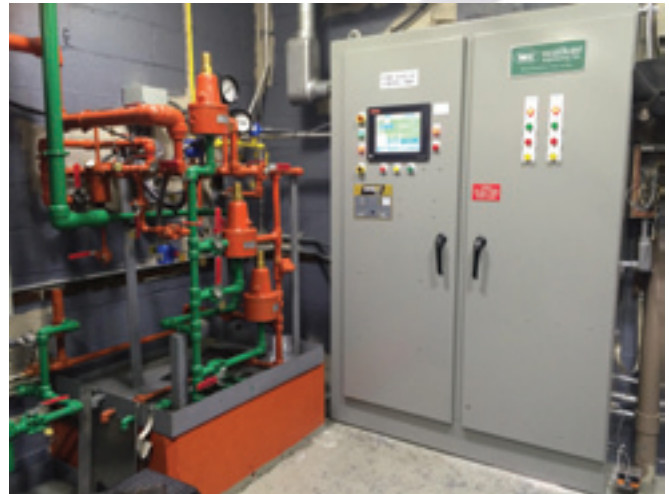
Above: A typical retrofit ladder. A pump house ladder allows control of feeder pressure through pressure relief valves, check valves and instrumentation.
