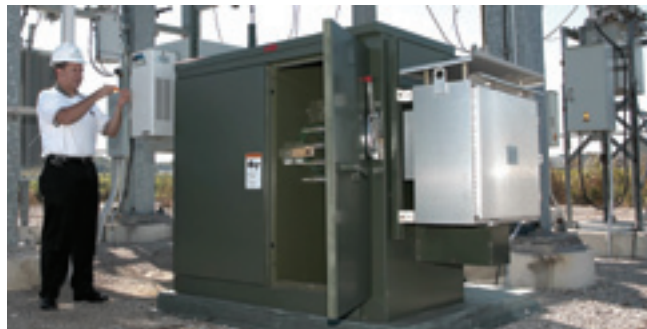
A power line communication system operates on existing power line infrastructure, with communications equipment required in the substation.
