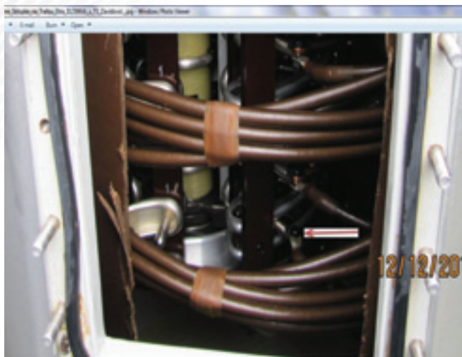
Figure 7. View of the selector through the manhole, loose bolt indicated
