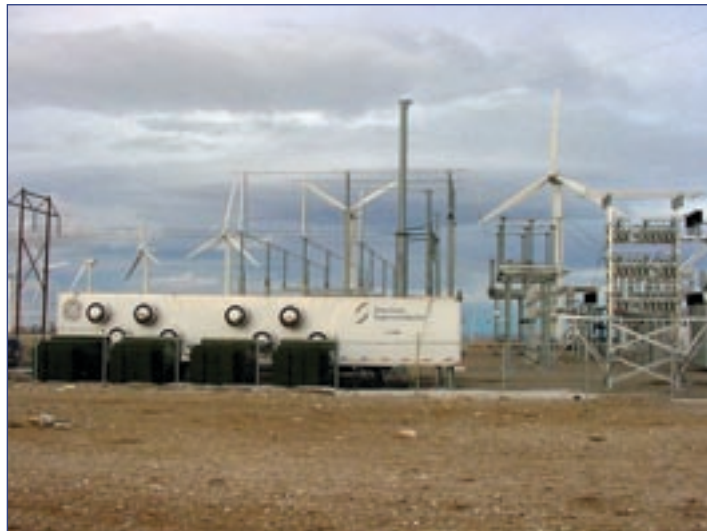
Figure 3: A D-VAR system providing complete voltage control and regulation at PacifiCorp's 135 MW wind farm in Foote Creek, Wyoming.
