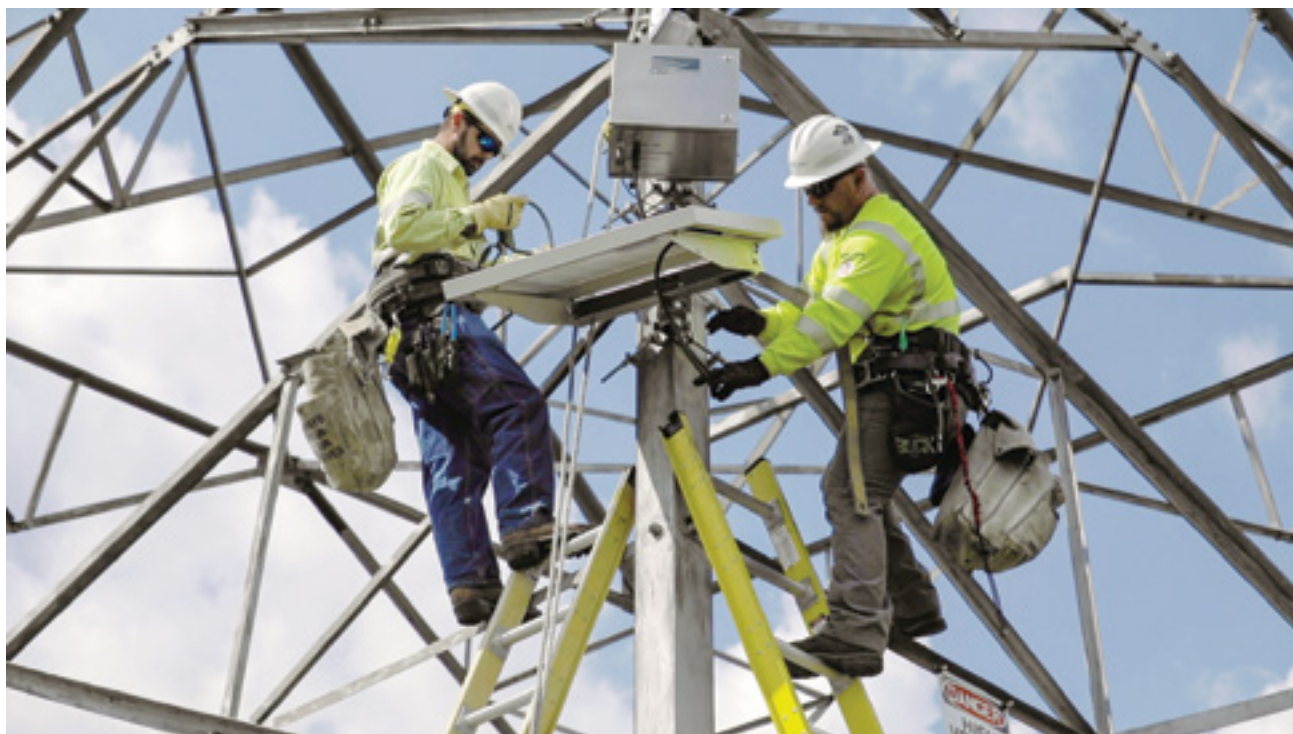
Lineworkers secure a LineVision non-contact sensor on an AES transmission tower. Source: LineVision.
