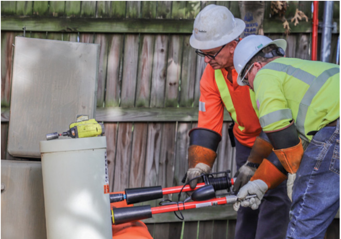
Upgrading legacy infrastructure with cable rejuvenation technologies helps extend lifespan and reduce capital outlay. Source: Southwire
