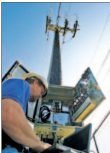
Distribution Management Pilot Power Control System Supervisor, Stephen Driskell, programs an air switch for a distribution management pilot program. Thirty-nine of the air switches and related equipment will be tested with a software system that enables the devices to communicate in real-time with Austin Energy's Energy Control Center.
