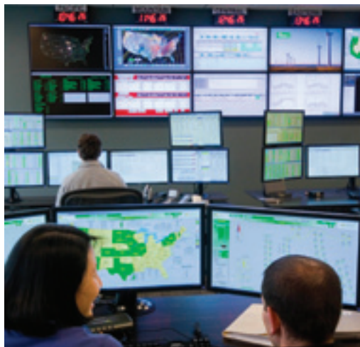
The National Control Center SCADA system monitors wind generation across 20 states
