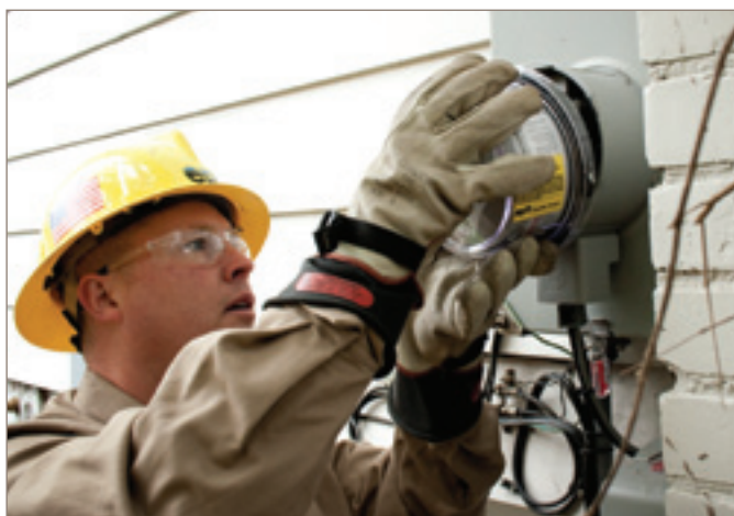
EPB technician deploys smart meter at customer home Photos courtesy of EPB
