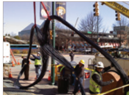
Fiber pull down in Chattanooga. EPB is building a lightning-fast, two-way fiber-optic network that will provide communications with every device in its distribution system.
