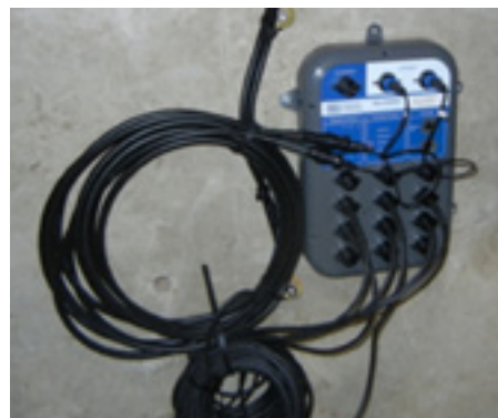
Fig 4: SEL Underground 8301A Faulted Circuit Indicator
