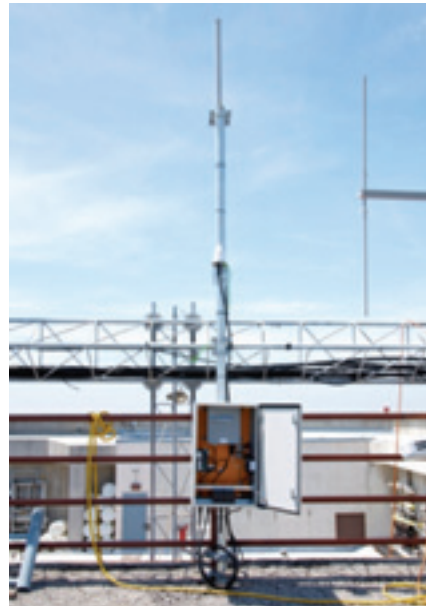
Fig 3: Antenna diversity shown for a manhole endpoint installation
