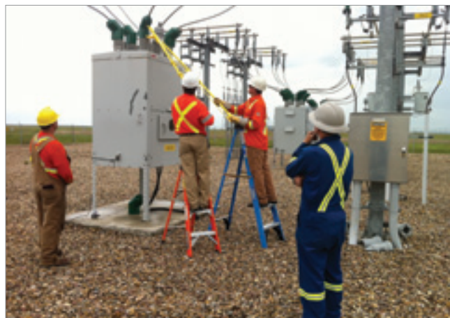
Figure 4: Energized installation using specialized hotline tools.
