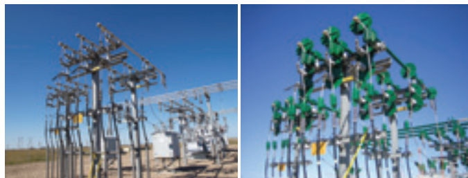
Figure 3: Low-voltage connections and equipment pre-and post coverup installation. The underground connectors, dropout switch bases, lightning arrestors, pipe bus, and breaker bushings are all covered.
