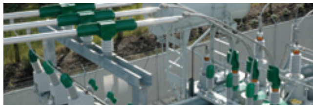
Figure 2: A typical custom cover-up installation using Greenjacket products
